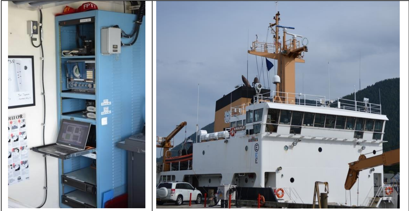
Figure B-14. (Left) Receiver and laptop mounted in rack in chart room on USCGC MAPLE. (Right) The HF receive antenna, located on starboard aft corner of bridge wing.
