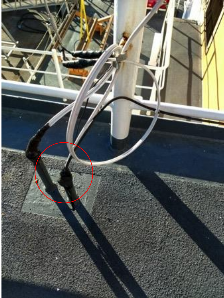
Figure B-12. Antenna cable run through existing stuffing tube.
